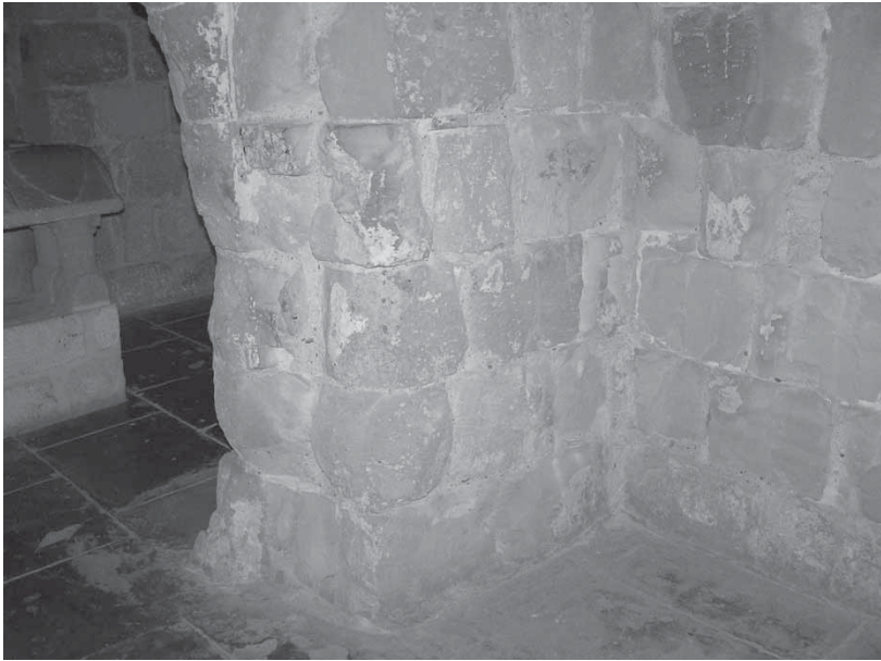
Fig. 27: Limassol Castle, lower level of cells, fire-damaged masonry [M. Olympios].
